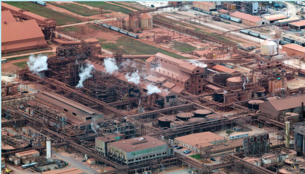
An aluminium production plant
