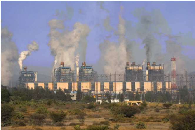
Oil refinery, Mexico
